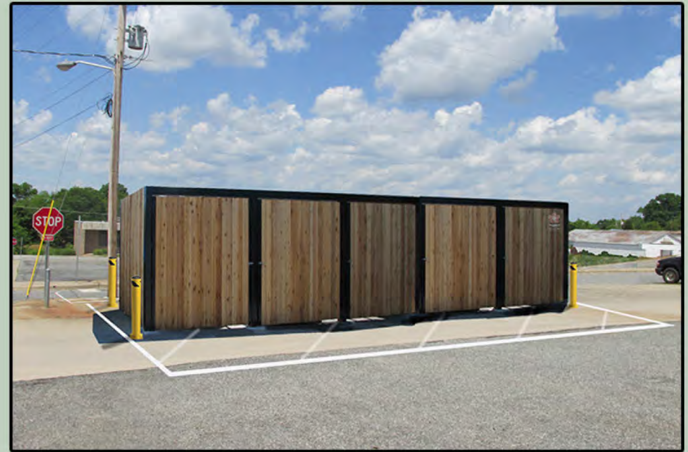
McDANIEL ALLEY DUMPSTERS AFTER
