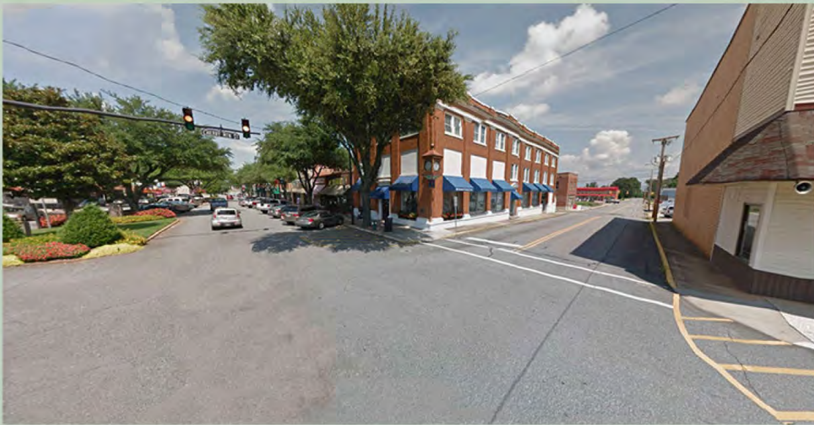
EAST MAIN STREET AT DEPOT STREET AND CHERRY MOUNTAIN STREET VIEW 2 BEFORE
