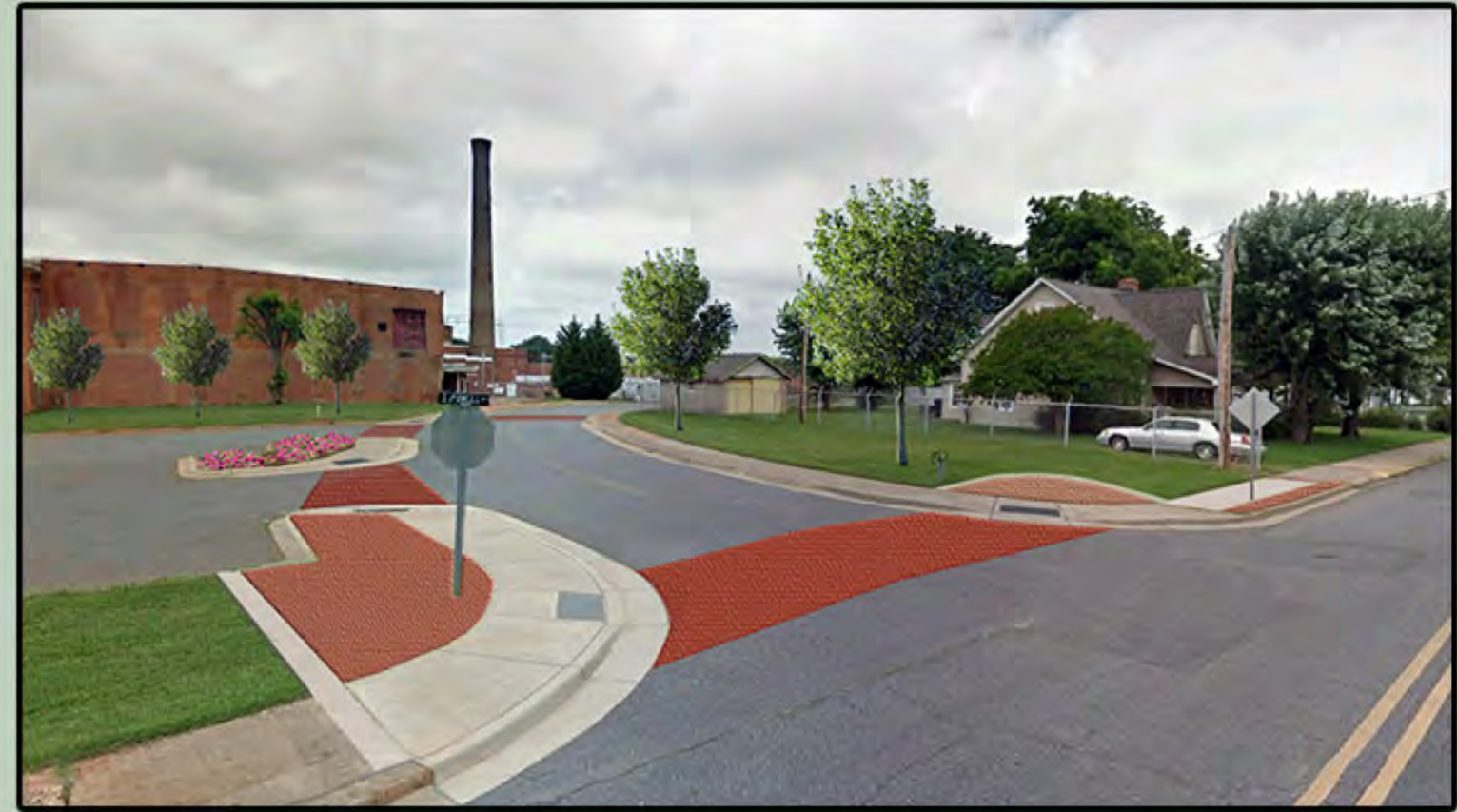
POWELL STREET & MILL STREET AFTER
