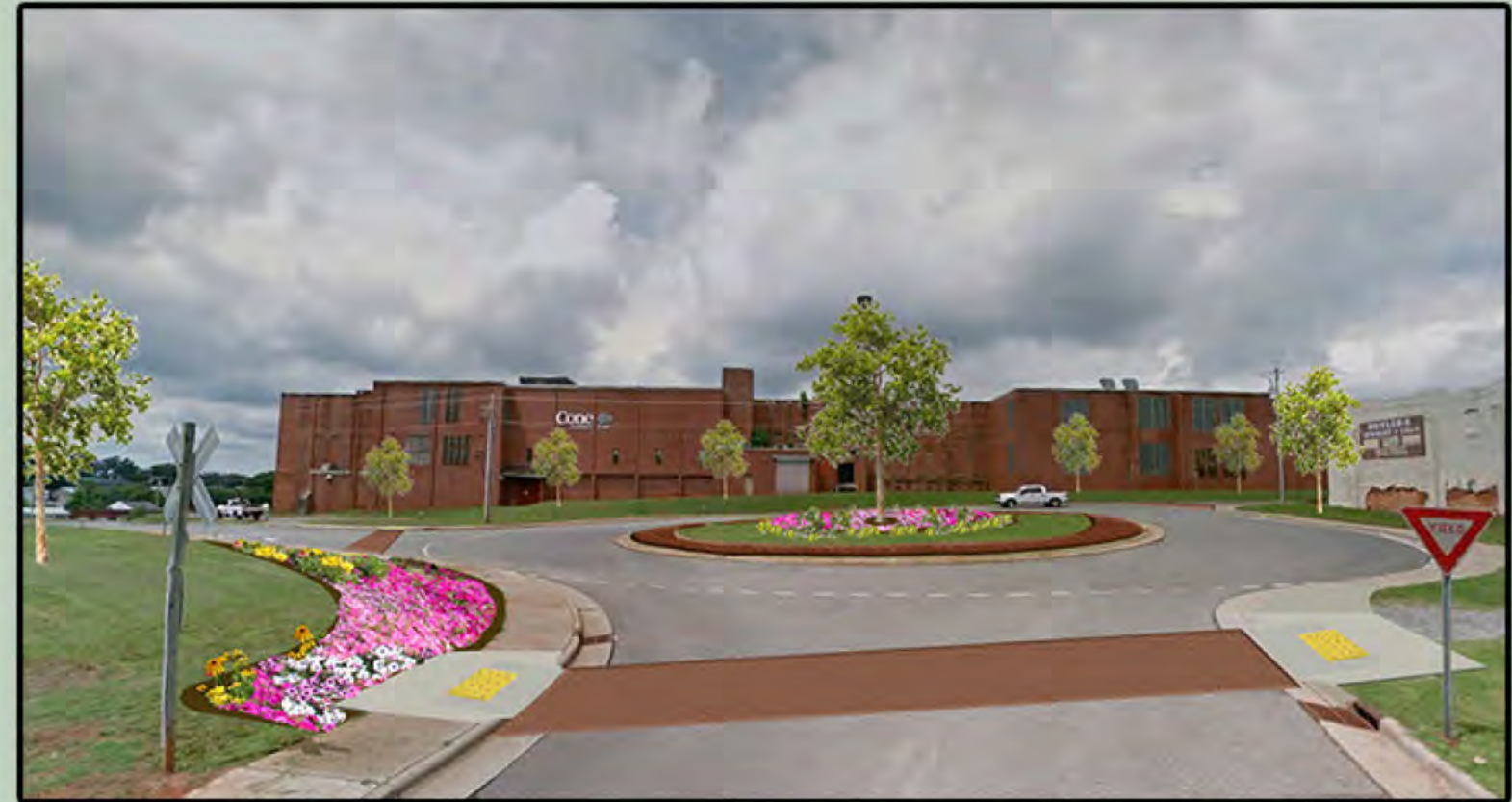
MILL STREET & HARMON STREET ROUNDABOUT AFTER
