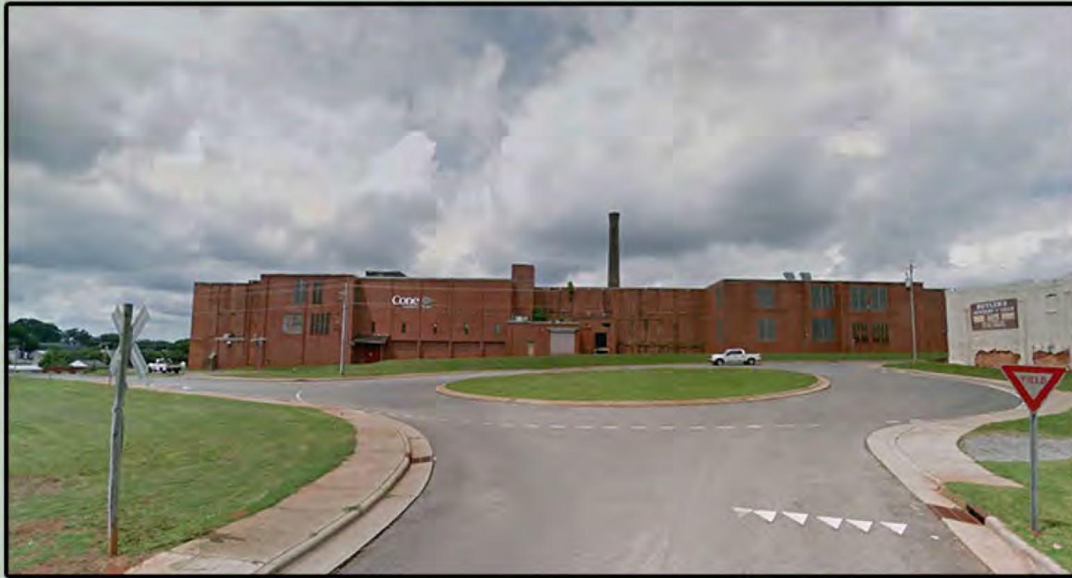
MILL STREET & HARMON STREET ROUNDABOUT BEFORE
