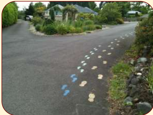
D: Pedestrian shared street markings in Olympia, WA.
