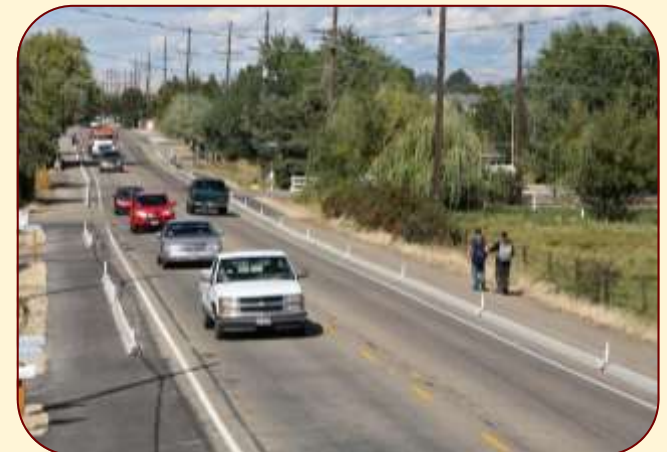
F: Shoulder/extruded curb pathway in Ada County, ID (constructed with federal Safe Routes to School funds)
